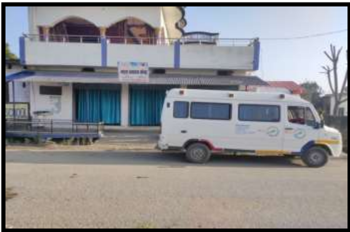
Mala Clinic, Village – Rampur, Sahaspur, Dehradun.
